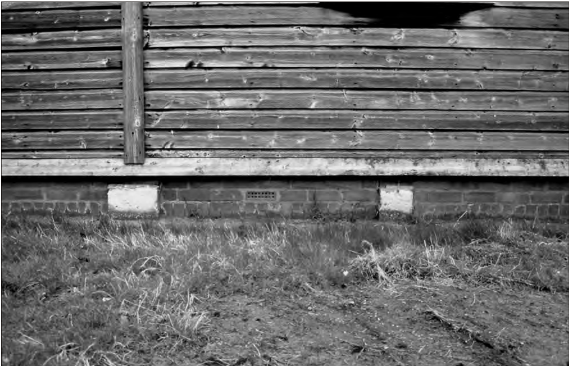
Plate 38 Saighton Camp, Chester: concrete foundation pillars evident in blocks 21, 22, 23 + 39
