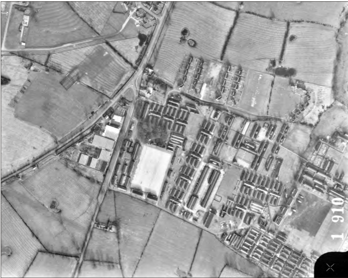
Plate 2a, Saughton Camp, Chester: 1970 aerial photograph
