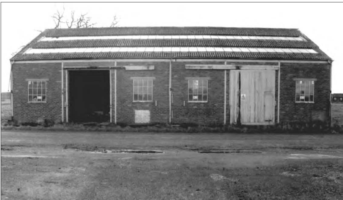
Plate 50 Saighton Camp, Chester: east facing elevation of building 43
