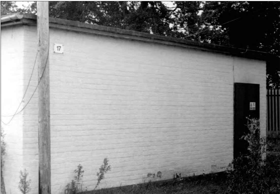
Plate 16 Saighton Camp, Chester: north facing elevation of building 17
