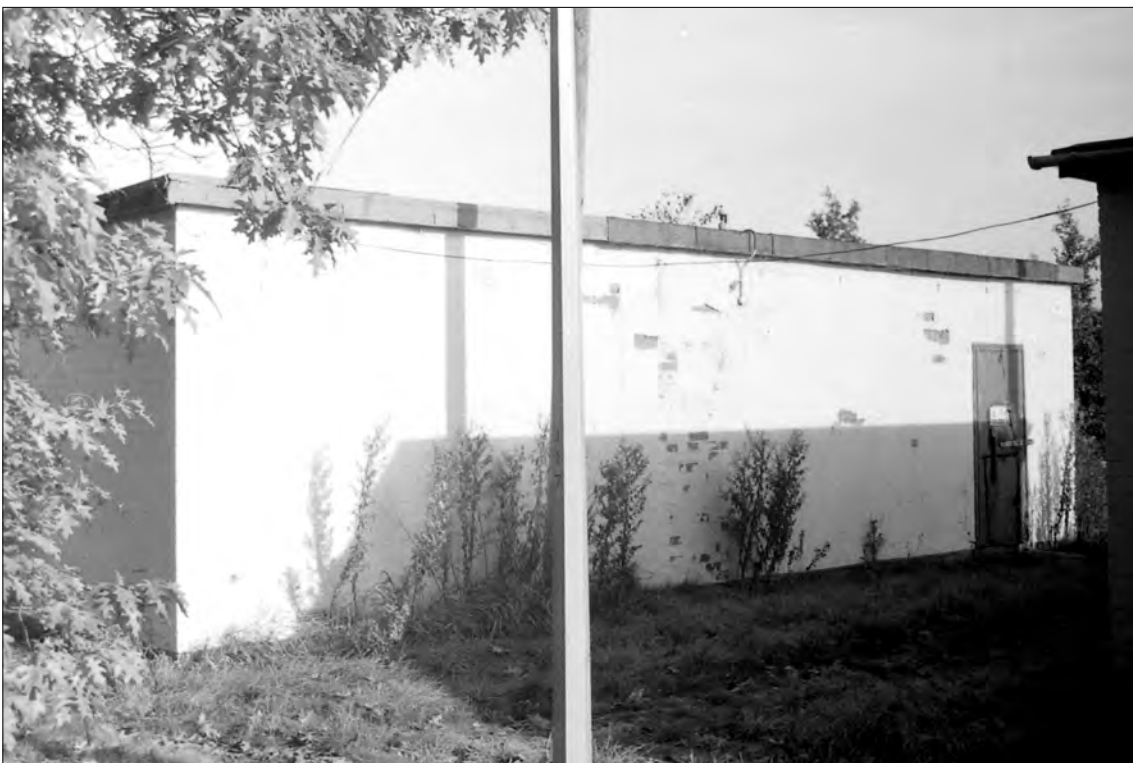
Plate 18 Saighton Camp, Chester: south facing elevation of building 18
