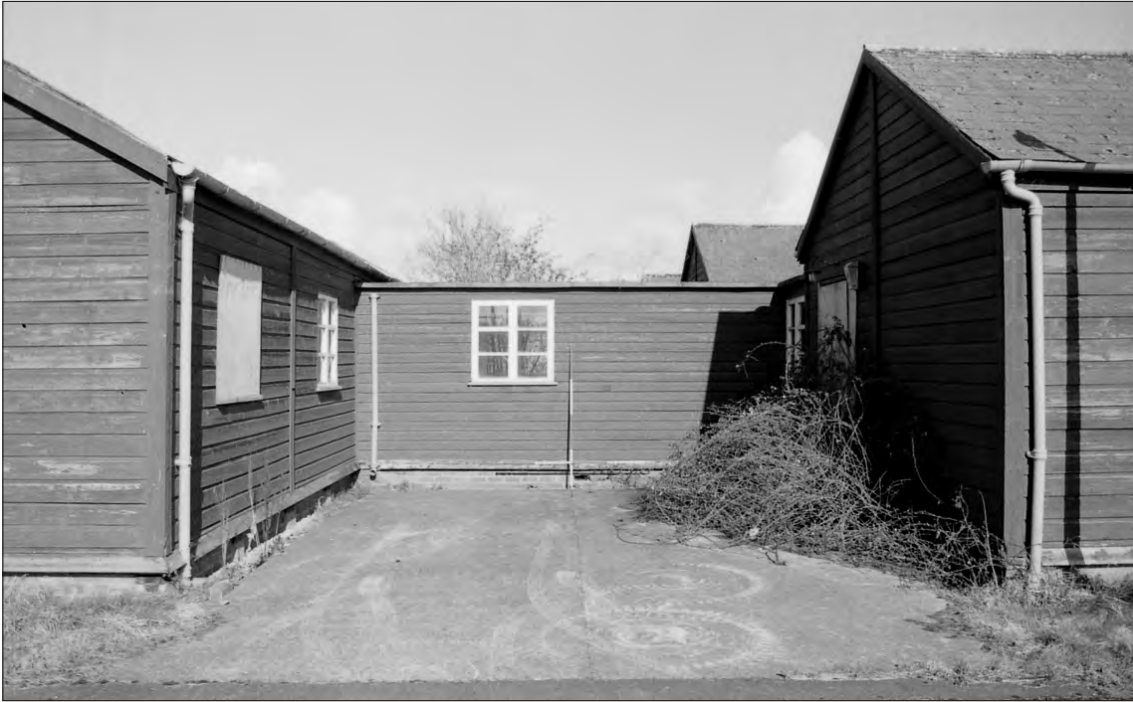
Plate 39 Saighton Camp, Chester: west facing elevation of south-western corridor of building 39
