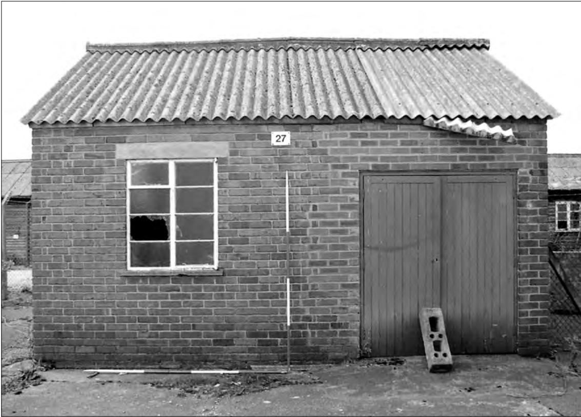
Plate 25 Saughton Camp, Chester: east facing elevation of building 27
