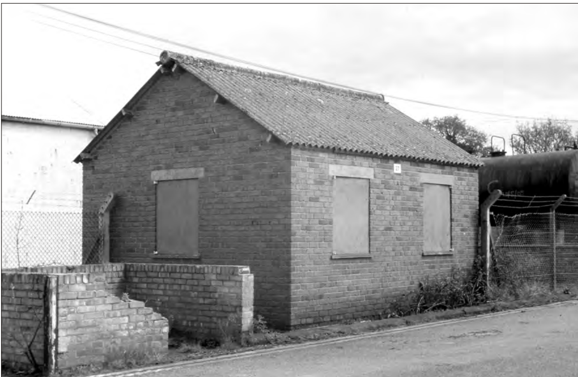
Plate 24 Saighton Camp, Chester: north and west facing elevations of building 27
