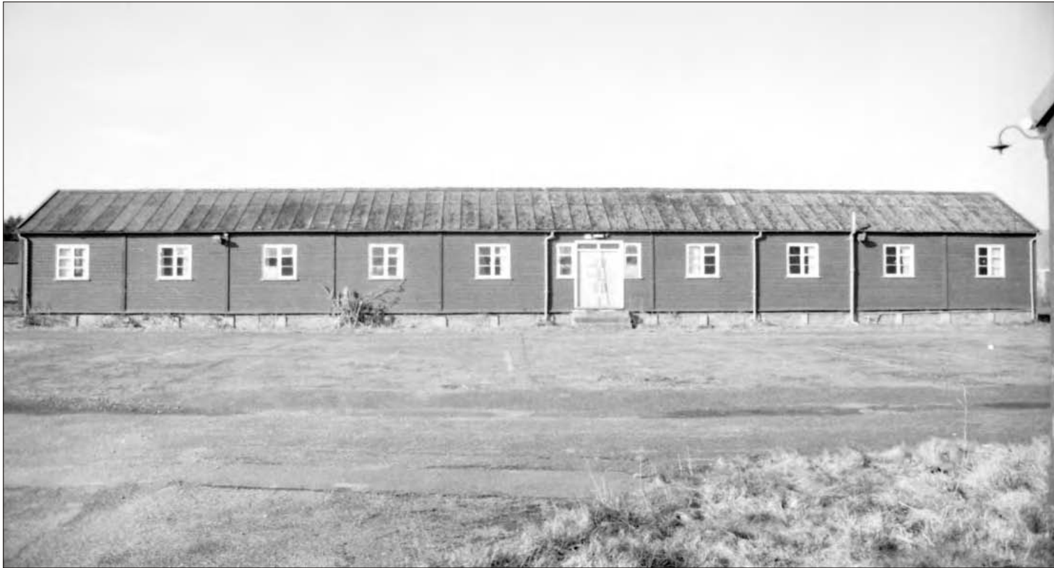
Plate 35 Saighton Camp, Chester: east facing elevation of building 35
