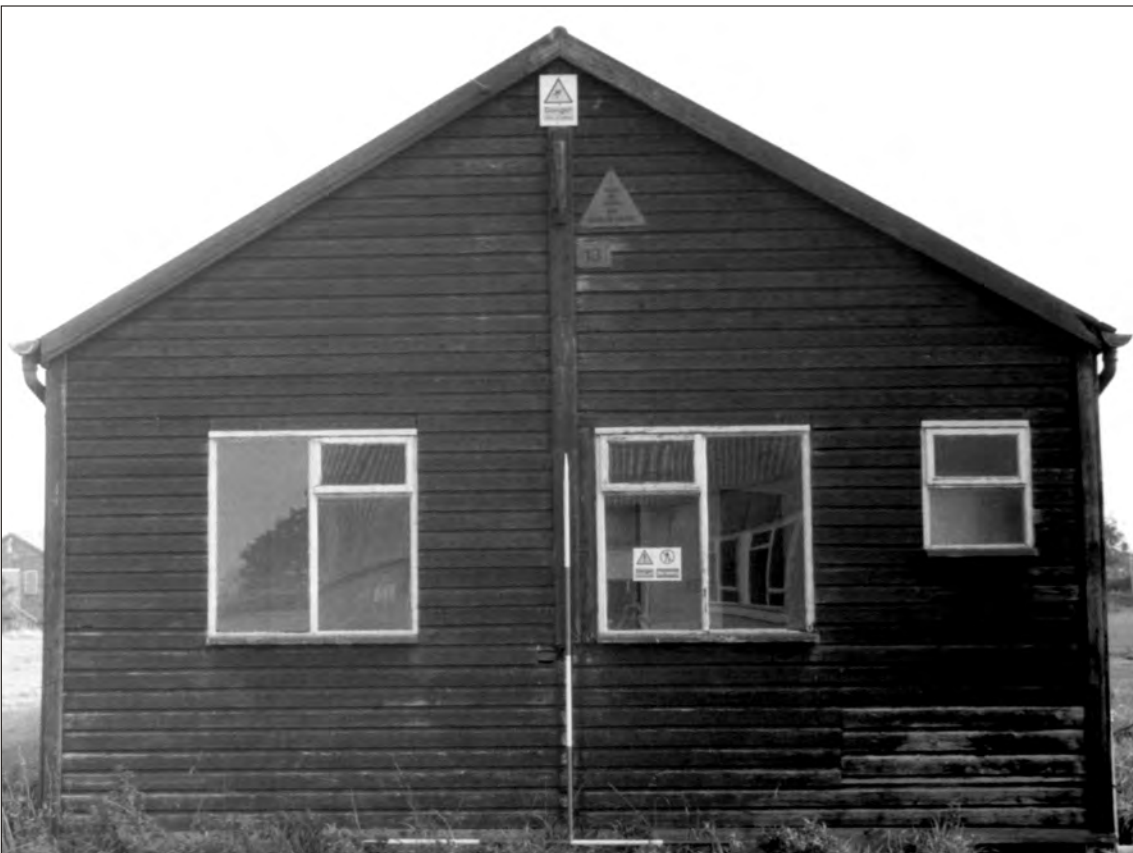
Plate 12 Saighton Camp, Chester: north facing elevation of building 13
