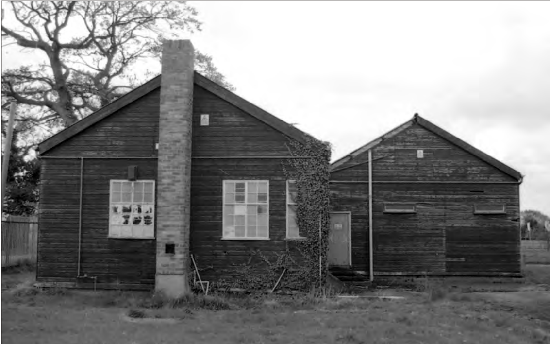
Plate 4 Saighton Camp, Chester: south facing elevation of building 4
