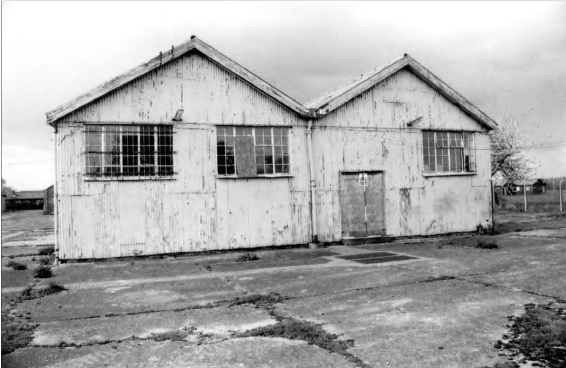
Plate 33 Saighton Camp, Chester: south facing elevation of building 30
