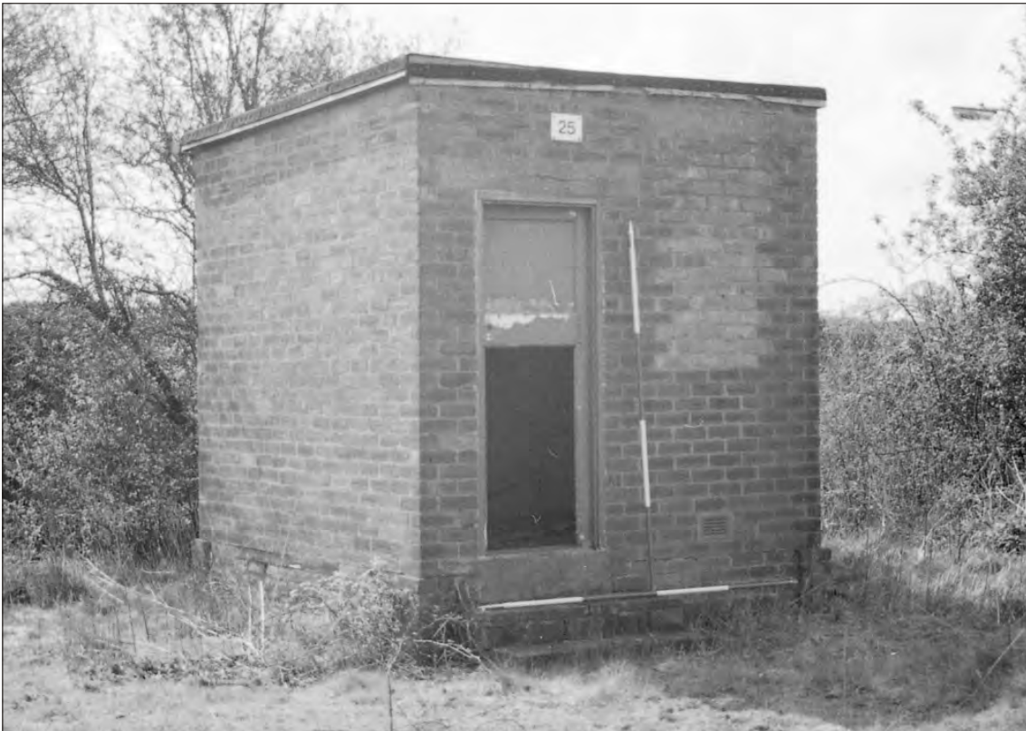
Plate 21 Saighton Camp, Chester: north and west facing elevations of building 25
