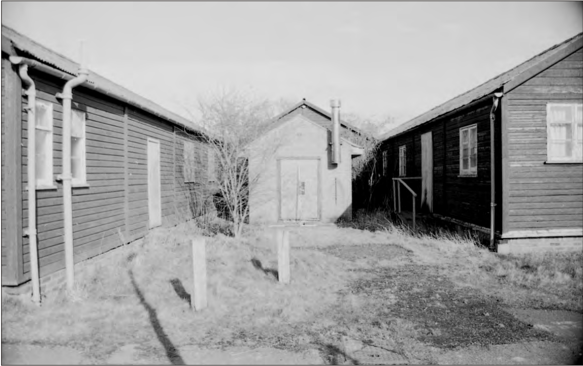
Plate 37 Saighton Camp, Chester: south facing elevation of boiler house, building 35
