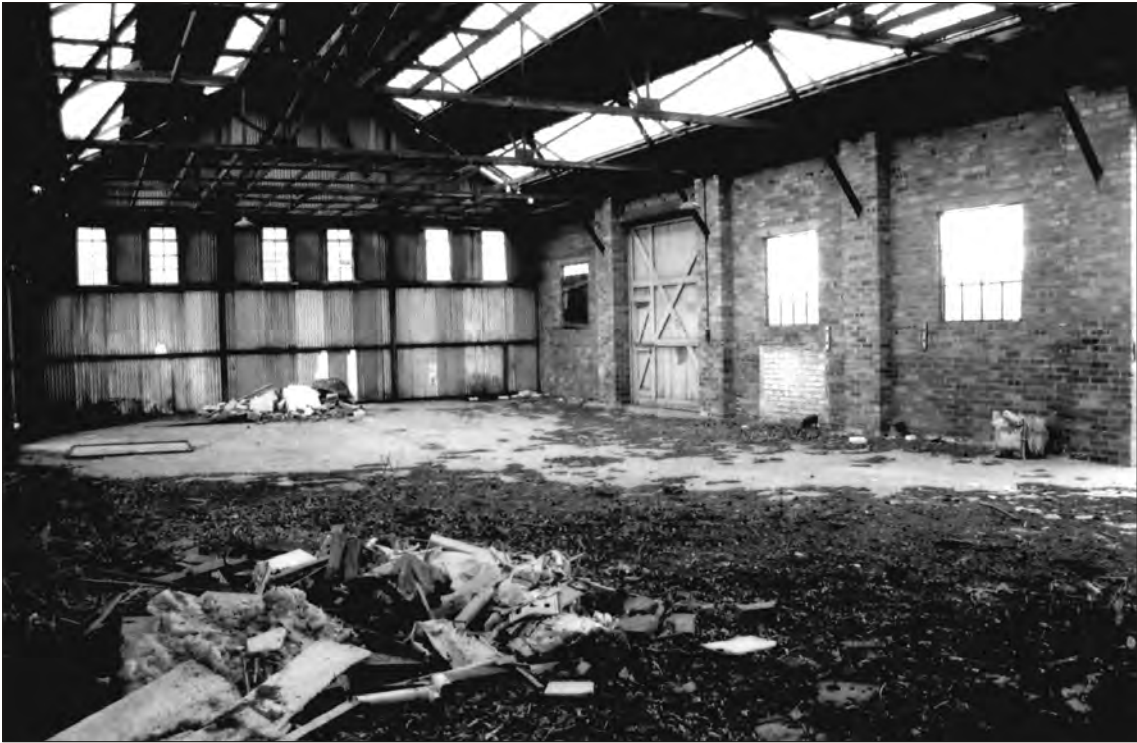
Plate 53 Saighton Camp, Chester: oblique shot of interior of building 43, looking north east
