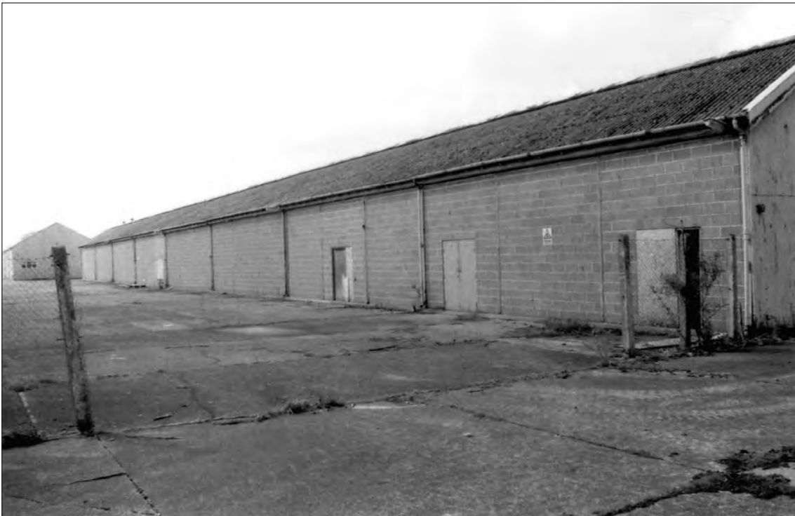
Plate 28 Saighton Camp, Chester: east facing elevation of building 29
