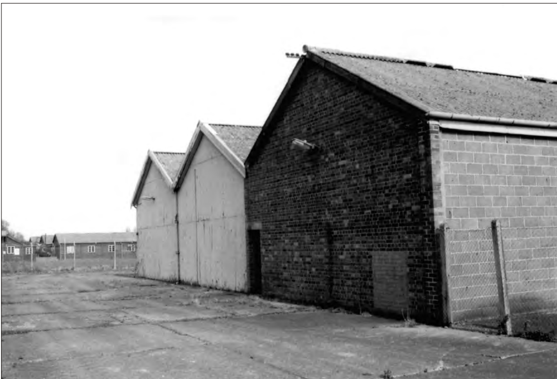
Plate 32 Saighton Camp, Chester: north facing elevation of building 30
