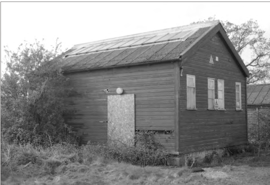
Plate 20 Saighton Camp, Chester: east facing elevation of building 24
