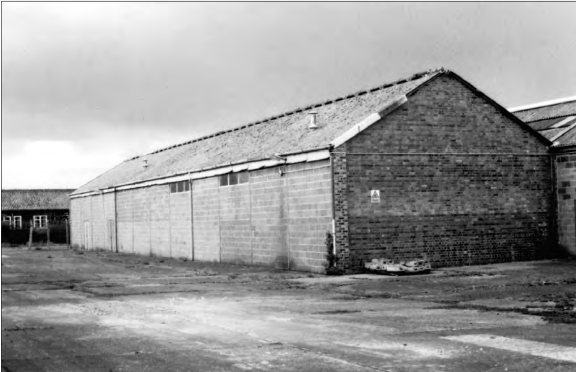
Plate 31 Saighton Camp, Chester: west facing elevation of western shed of building 30
