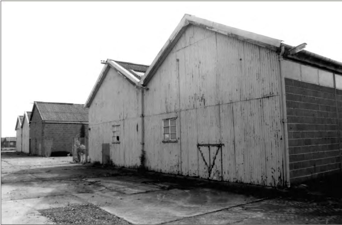
Plate 29 Saighton Camp, Chester: north facing elevation of building 29
