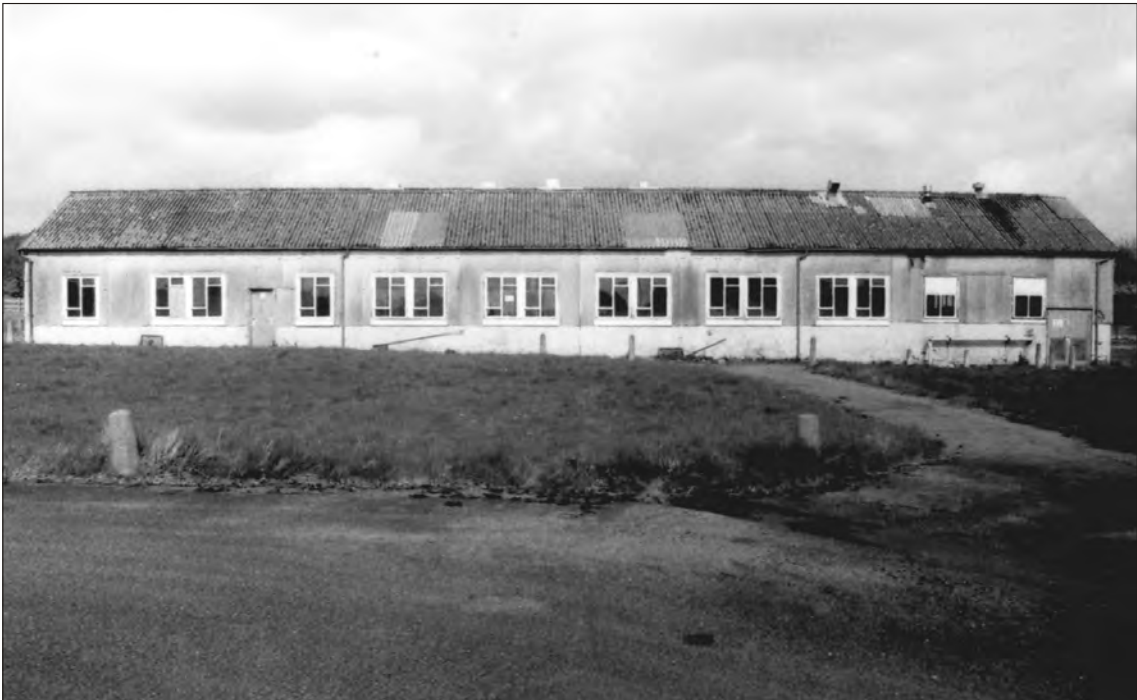
Plate 14 Saighton Camp, Chester: south facing elevation of building 15
