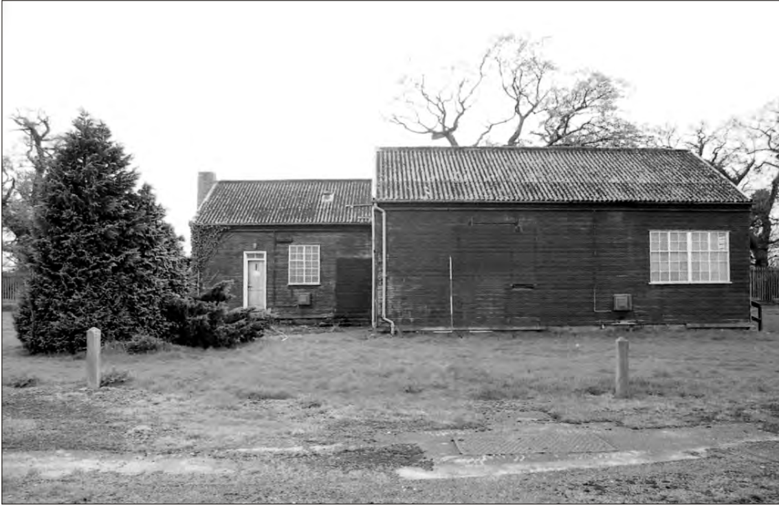
Plate 3 Saighton Camp, Chester: east facing elevation of building 4
