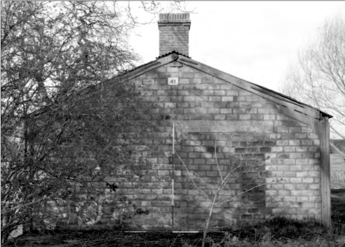
Plate 47 Saighton Camp, Chester: south facing elevation of building 41
