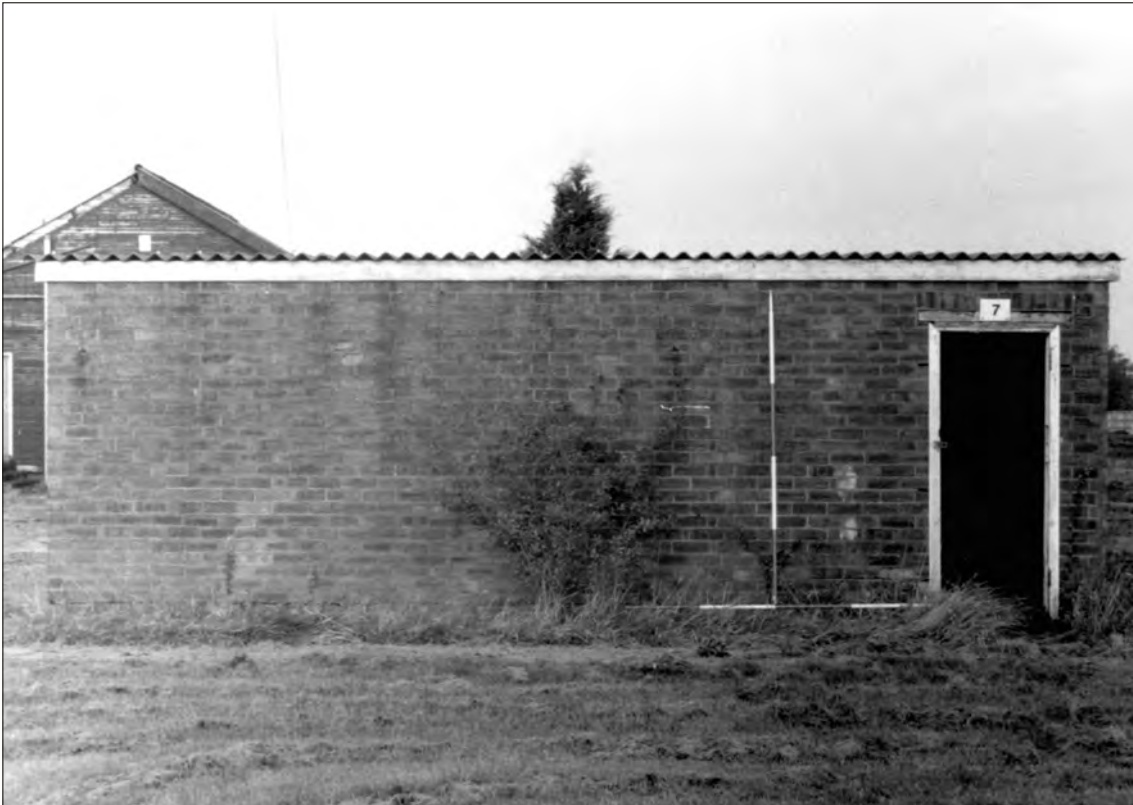
Plate 7 Saighton Camp, Chester: south facing elevation of building 7
