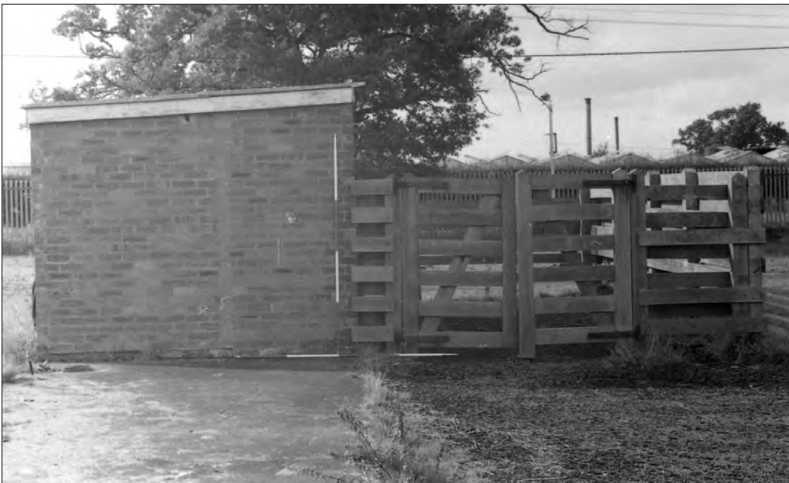
Plate 8 Saighton Camp, Chester: east facing elevation of building 7
