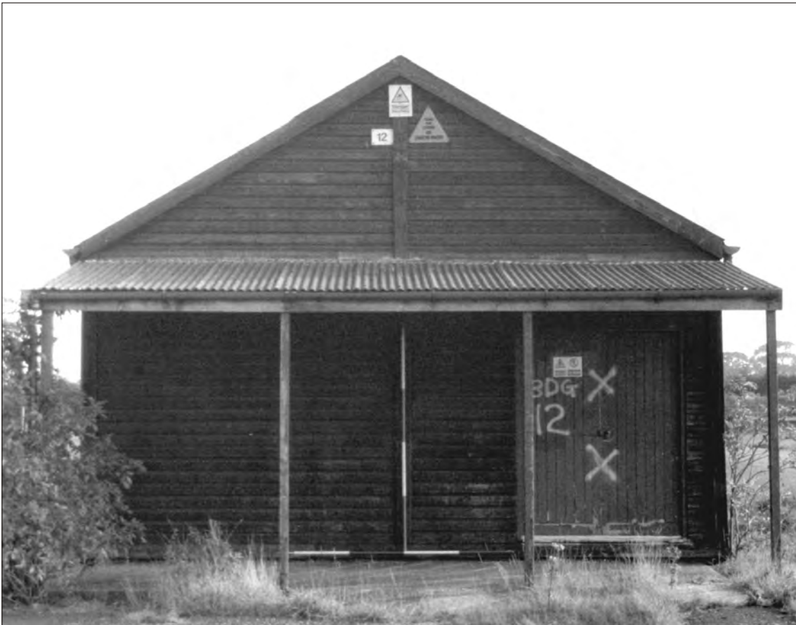
Plate 11 Saighton Camp, Chester: north facing elevation of building 12
