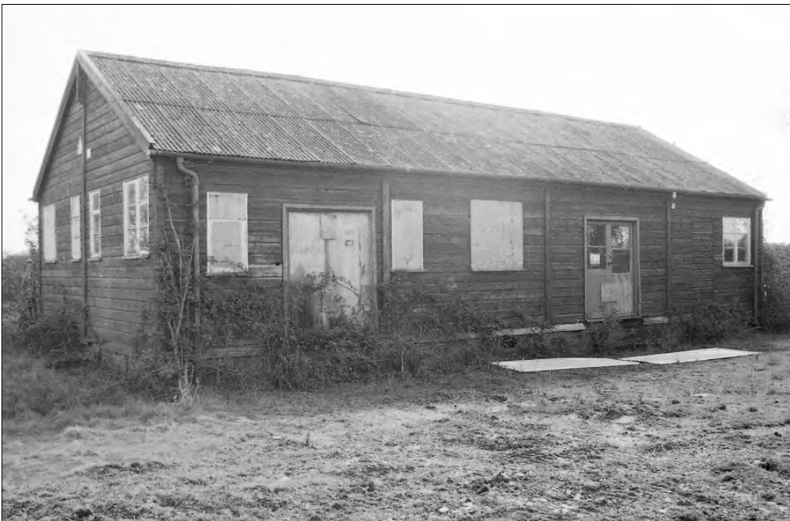
Plate 22 Saighton Camp, Chester: north and west facing elevations of building 26
