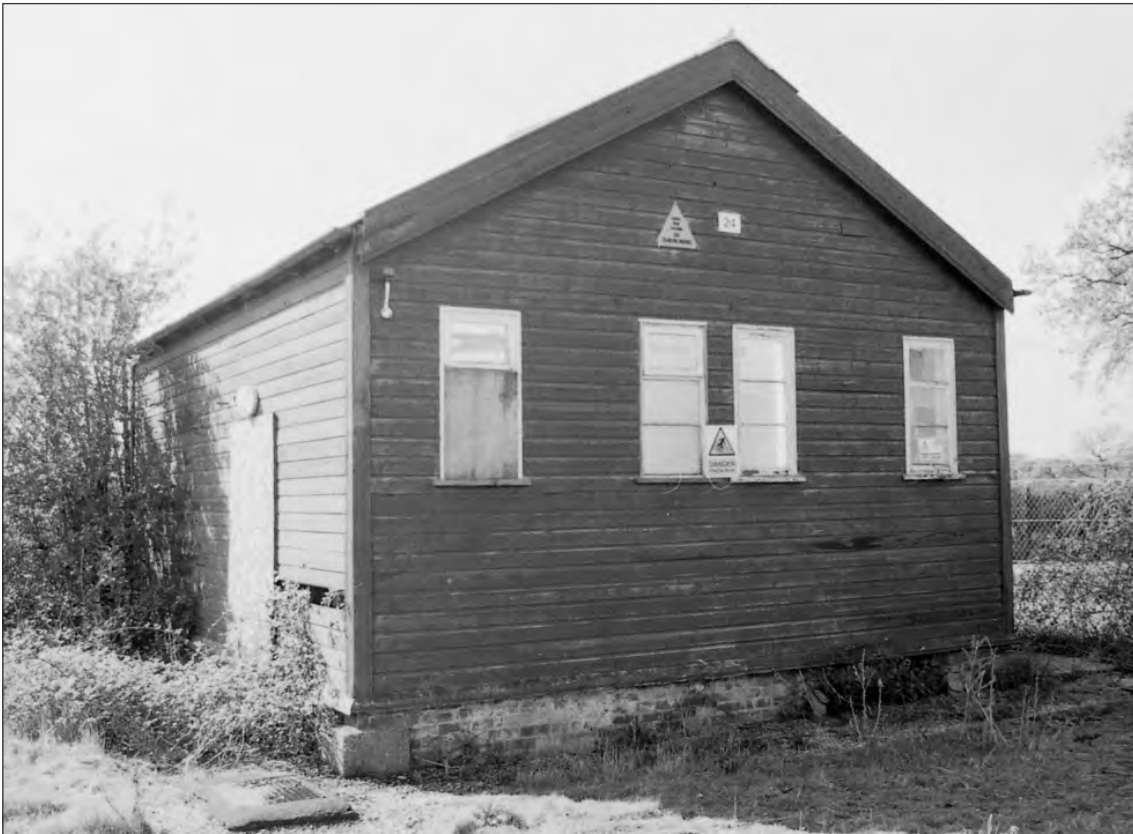
Plate 19 Saighton Camp, Chester: north facing elevation of building 24
