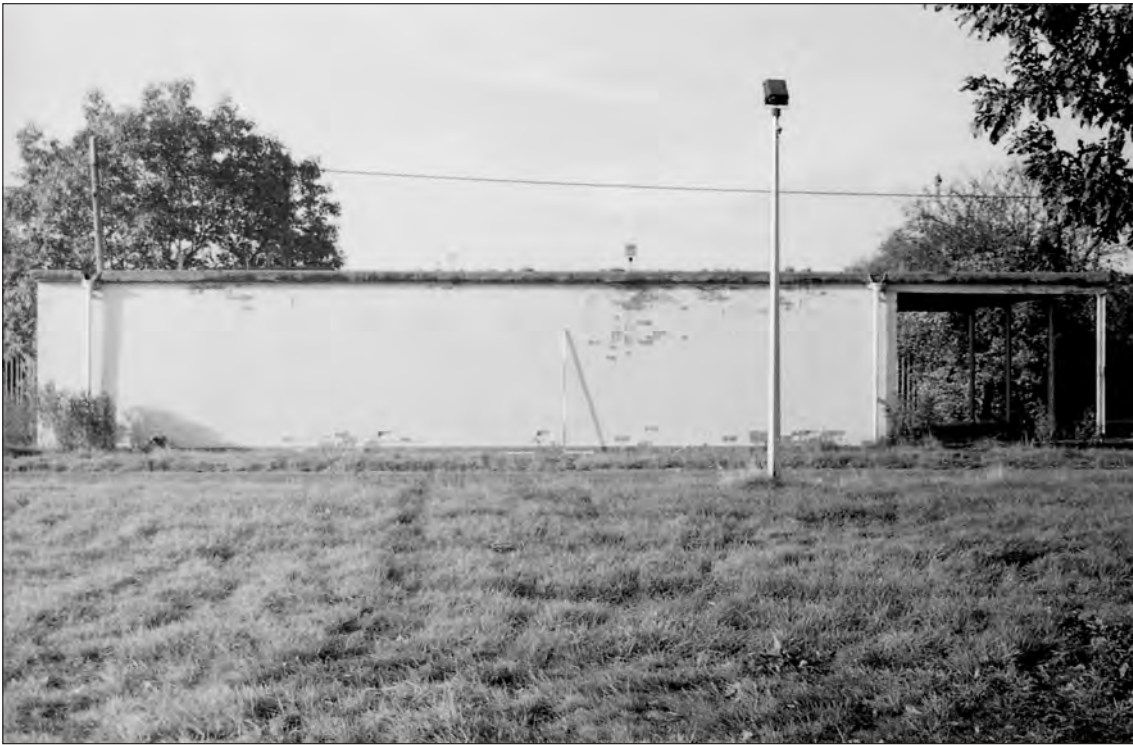
Plate 17 Saighton Camp, Chester: east facing elevation of building 18
