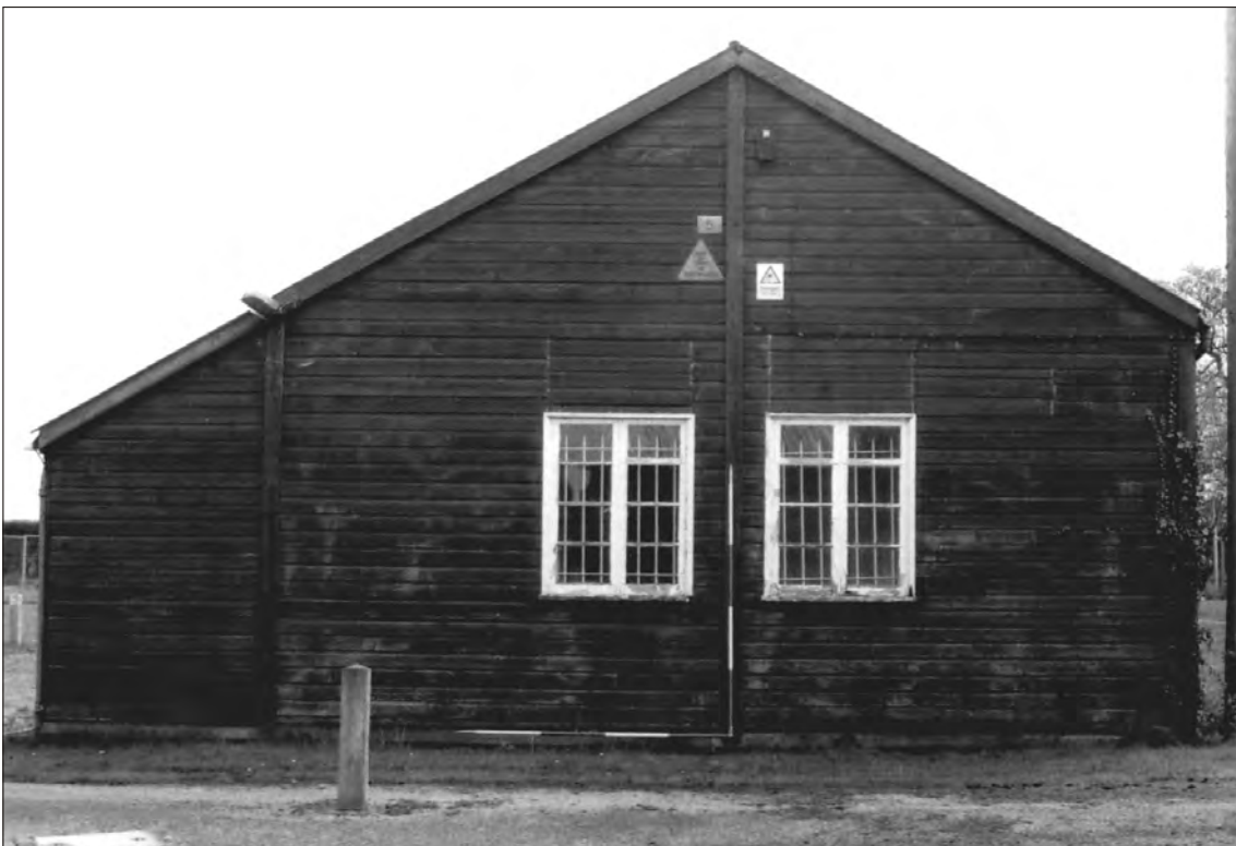
Plate 6 Saighton Camp, Chester: north facing elevation of building 5
