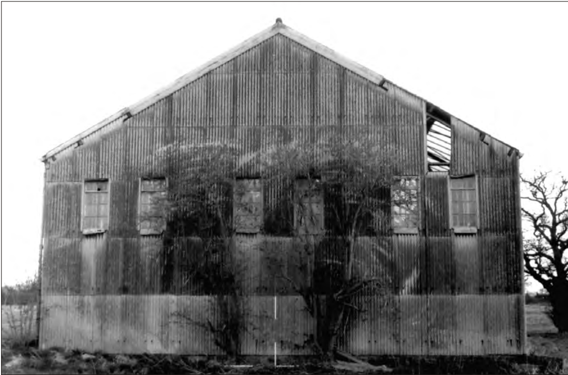
Plate 51 Saighton Camp, Chester: north facing elevation of building 42
