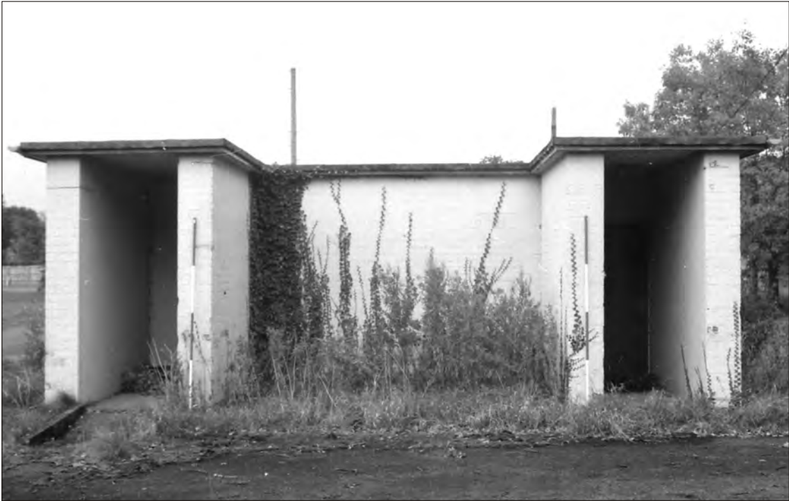
Plate 15 Saighton Camp, Chester: south facing elevation of building 17
