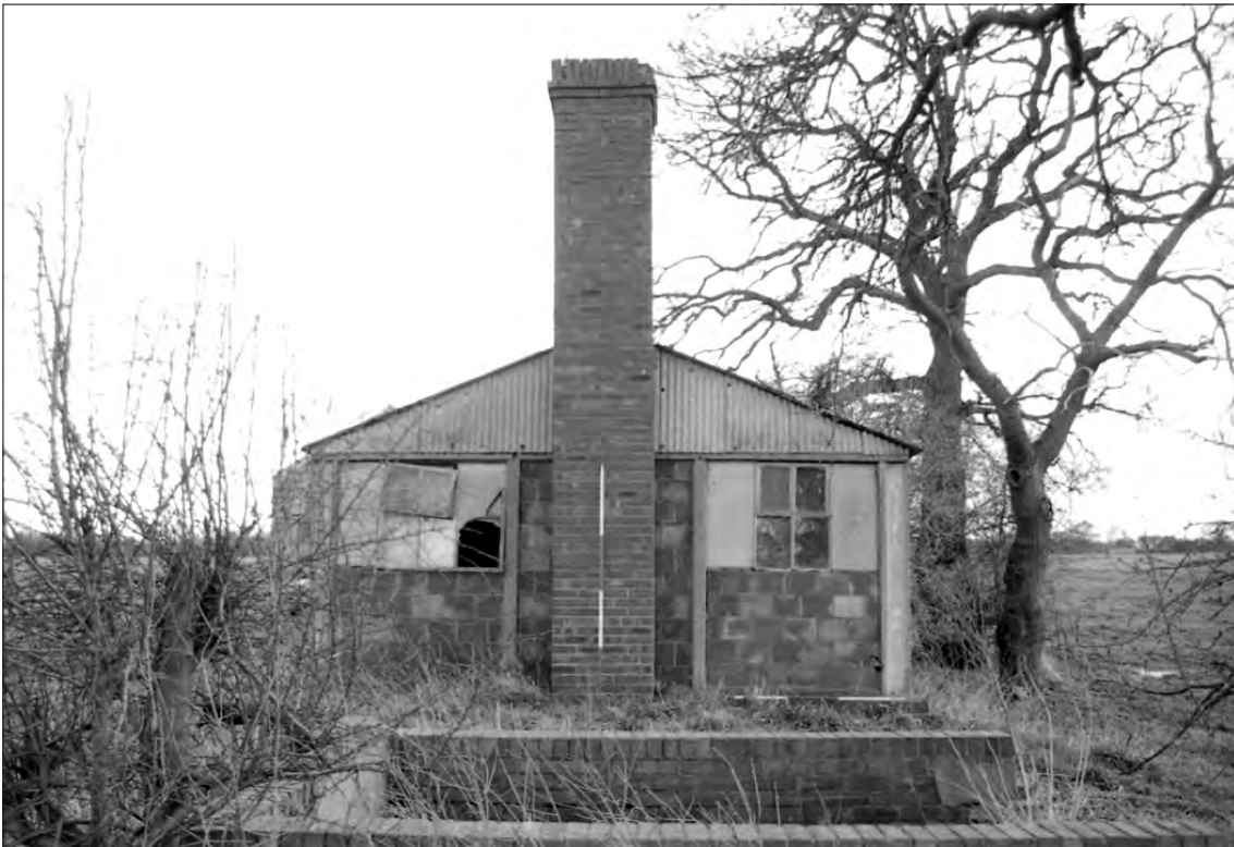
Plate 49 Saighton Camp, Chester: north facing elevation of building 41
