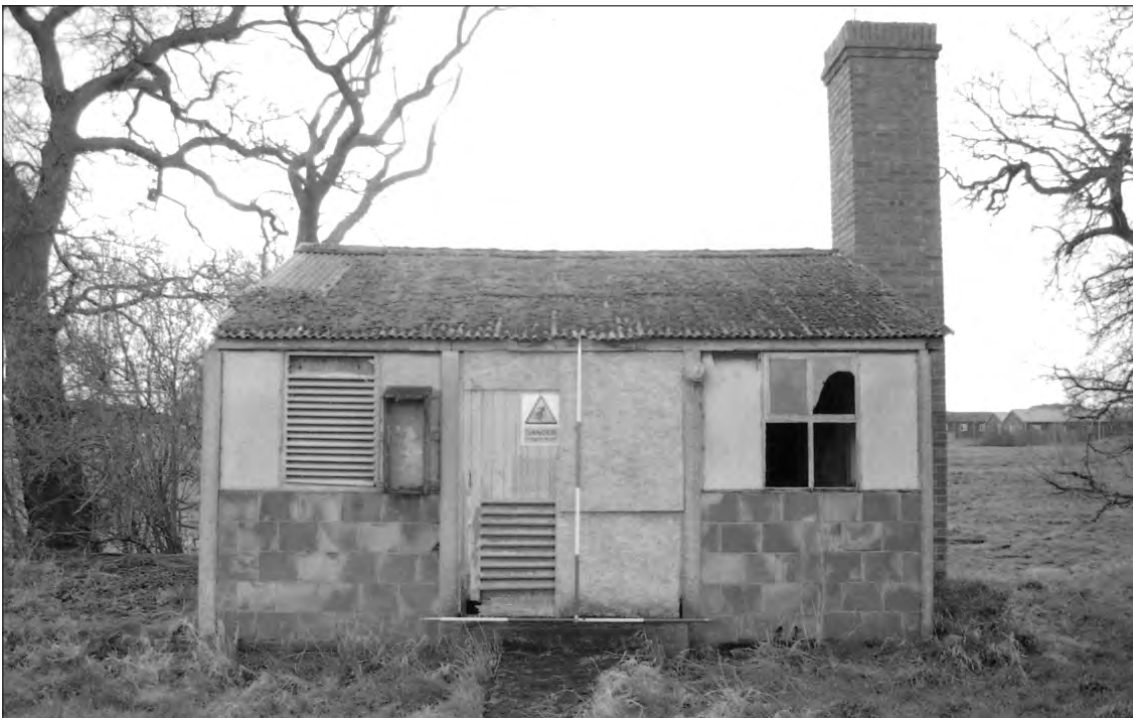
Plate 48 Saighton Camp, Chester: east facing elevation of building 41
