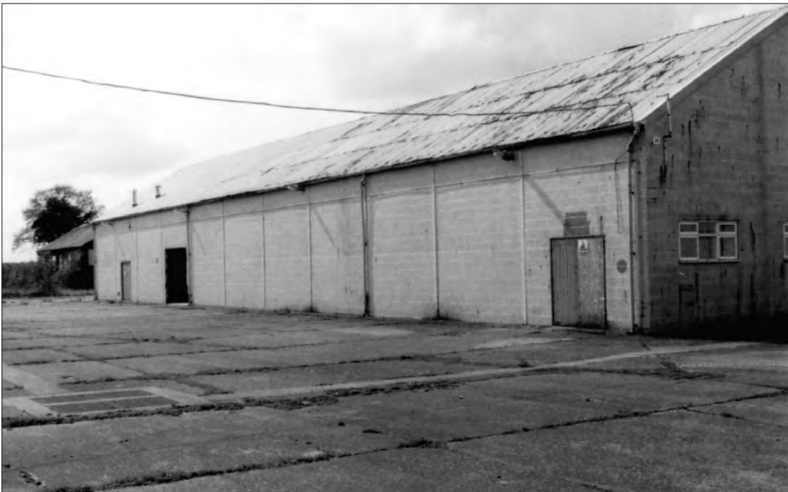
Plate 26 Saughton Camp, Chester: east facing elevation of building 28
