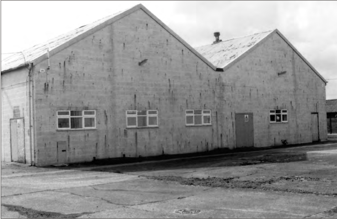
Plate 27 Saighton Camp, Chester: north facing elevation of building 28
