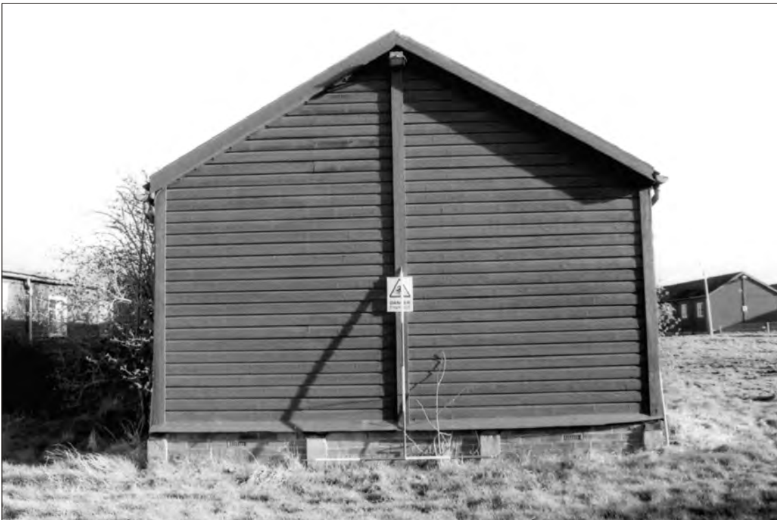
Plate 34 Saighton Camp, Chester: north facing elevation of building 35
